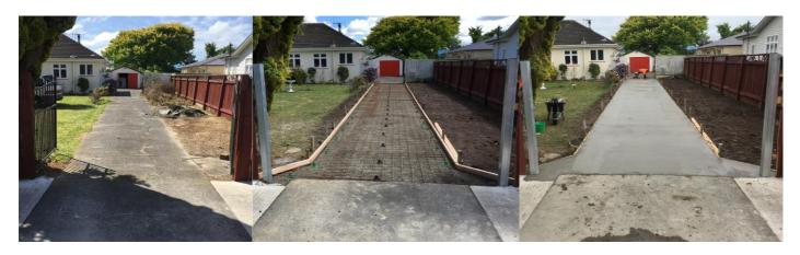
To prepare the site, we demolish any existing concrete, excavate the sub-soil and dump or recycle the spoil. Any drains are installed in trenches. We mark and box the edges, then level and compact a base of road metal to prevent the driveway from slumping or buckling. We lay steel mesh, tied together and stood up on "chairs" to ensure that it is suspended in the concrete to prevent cracking or splitting. Expansion joints are marked and set out.
